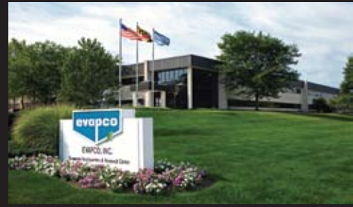
EVAPCO World Headquarters - Taneytown, Maryland, USA
