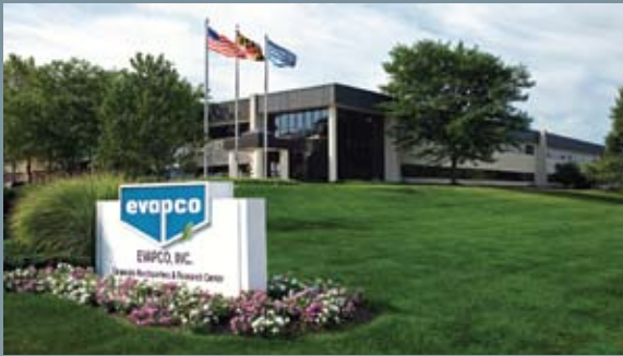
EVAPCO World Headquarters - Taneytown, Maryland, USA
